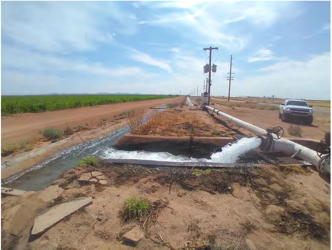
Figure 1. Groundwater being pumped to an irrigation canal to supply field crops in Central Arizona. Source: Simone A. Williams
