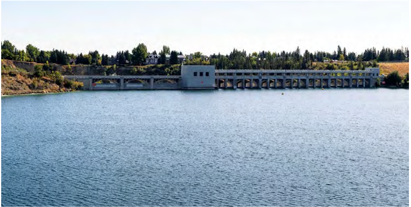
Glenmore Dam improvements mean less flooding and more drinking water for Calgary residents. Source: City of Calgary
